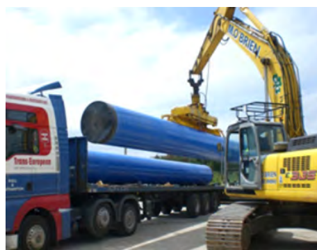
PIPE LENGTHS BEING UNLOADED USING A VACUUM LIFT
