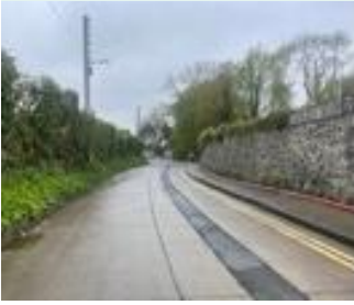
Outlet host on route to second hydrant
