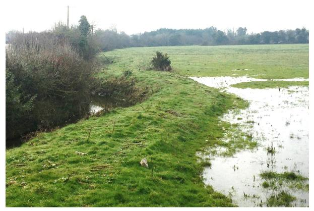
A low earthen bund or bank reducing or preventing overland flow entering the watercourse. (Photo: SMARTER\_BufferZ project)
