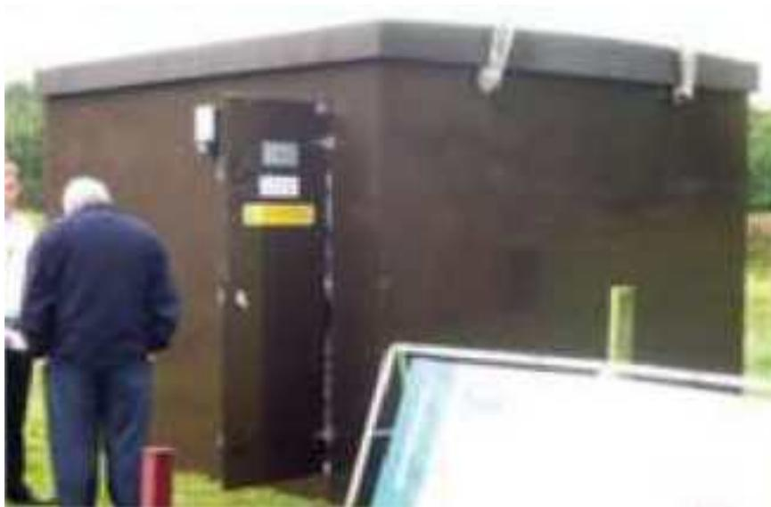
Figure 5 Typical orthophosphate dosing unit
