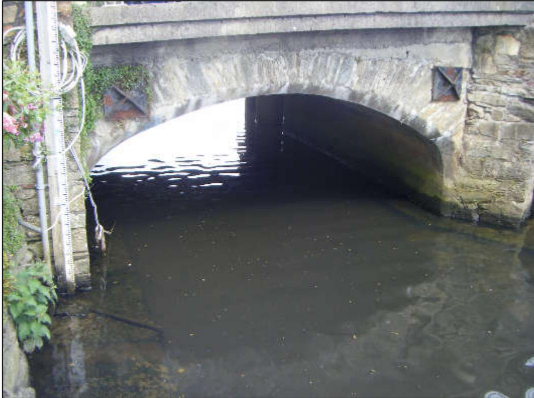
**Figure 13** View of the southernmost span of Arklow Bridge (note the concrete encasement around the west abutment)
